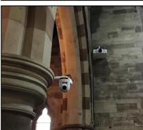
A Christie LW-751i 7,500 lumen projector for the main central screen and Sony SRG-300HW full HD motorised PTZ camera for projection, recording and online streaming.
